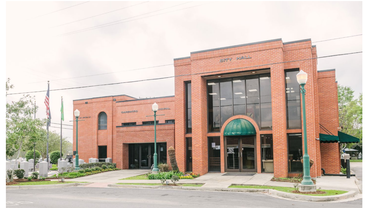
City Hall Source: DK Hebert Photography
