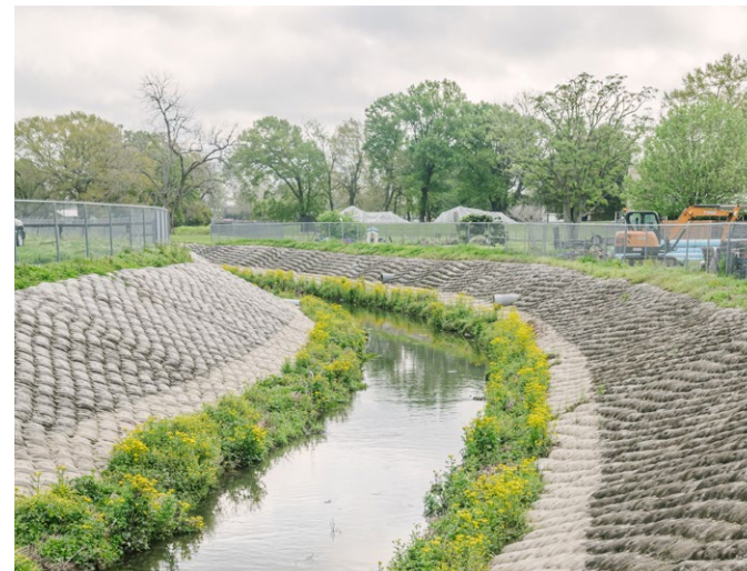
Existing Drainage System Source: DK Hebert Photography
