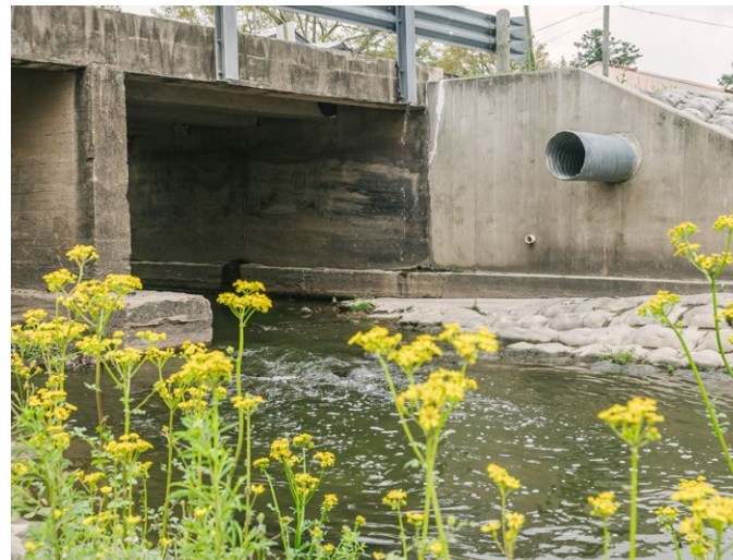
Existing Drainage System Source: DK Hebert Photography
